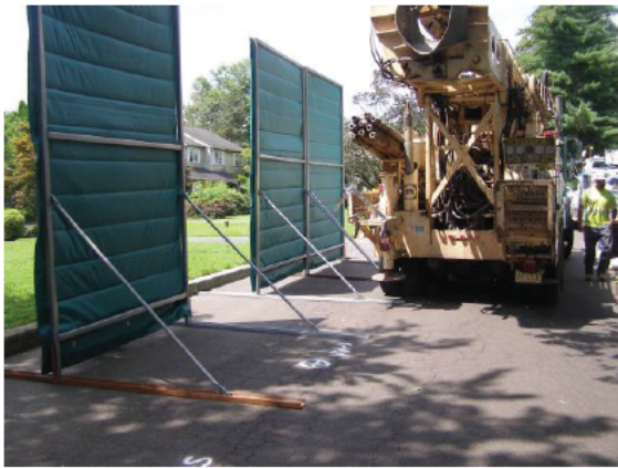
Sound barriers between drill rig and [redacted] 7-24-25 @ 11:50
