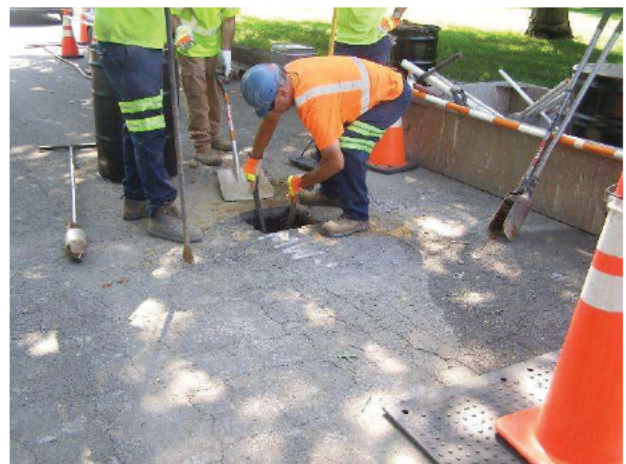
Photo 4: Hand digging prior to drilling
