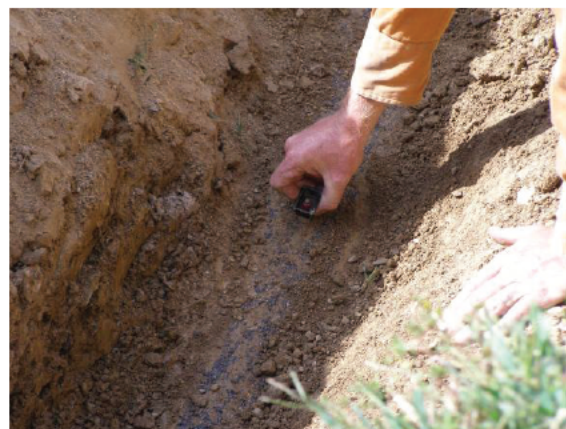
Magnetic tool used to locate the weld 9-29-25 @ 11:11
