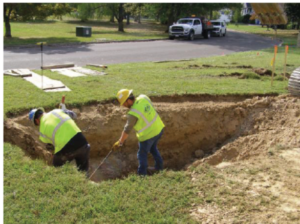
Hand clearing around pipeline with shovels 9-29-25 @ 11:08
