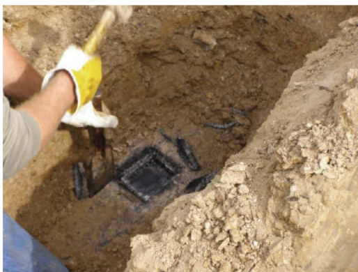
Weld in pipe located and coating removed 9-29-25 @10:34
