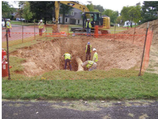
Orange snow fence set up around excavation 9-29-25 @ 14:48
