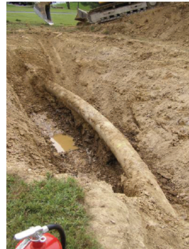
Uncovered pipeline from weld to areas of identified anomalies 9-29-25 @ 14:26
