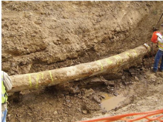
Anomaly locations marked with yellow paint 9-29-25 @ 14:48
