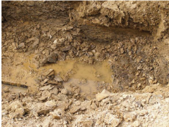
Water in excavation, no sheen or odor noticed 9-29-25 @ 14:23
