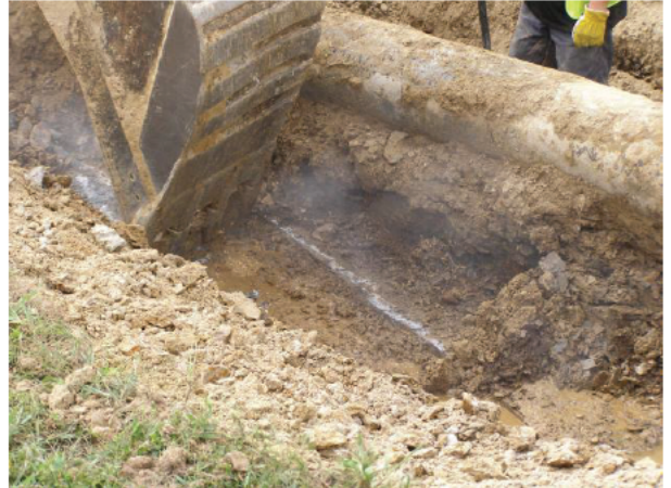
Bedrock encountered in excavation, approximately 7.5 feet bgs. 9-29-25 @ 13:46
