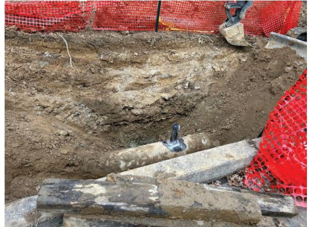
End of pipe flush - across from 140 Glenwood Ave. 2-4-25
