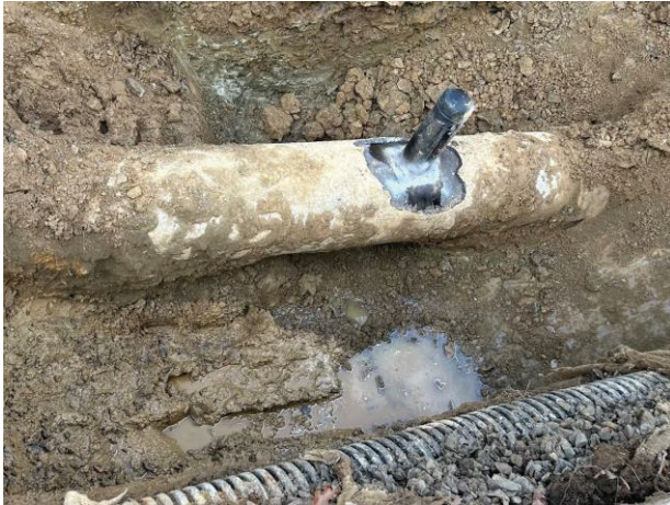
Groundwater in excavation across from 140 Glenwood Dr. 2-4-25
