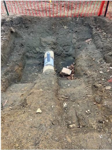
Input for pipe flush - across from 140 Walker Rd. 2-4-25
