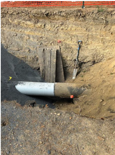
repaired pipeline near 121 Glenwood Ave. 2-4-25
