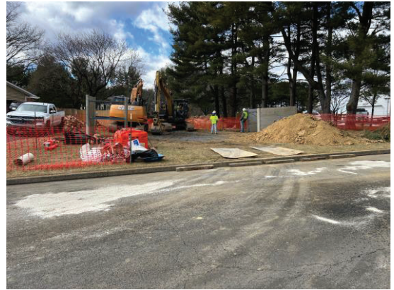
Location of repaired pipe next to 121 Glenwood Ave. 2-4-25
