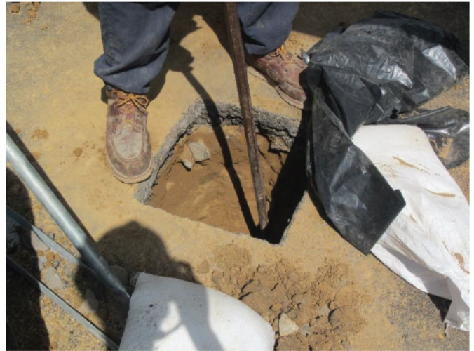
Hand clearing of Well C.
