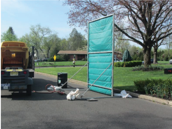
Sound barrier setup at Well B location prior to hand clearing.
