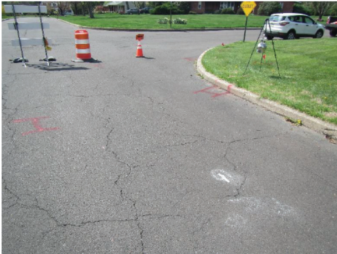
Re-marked underground utilities in the vicinity of Well C.
