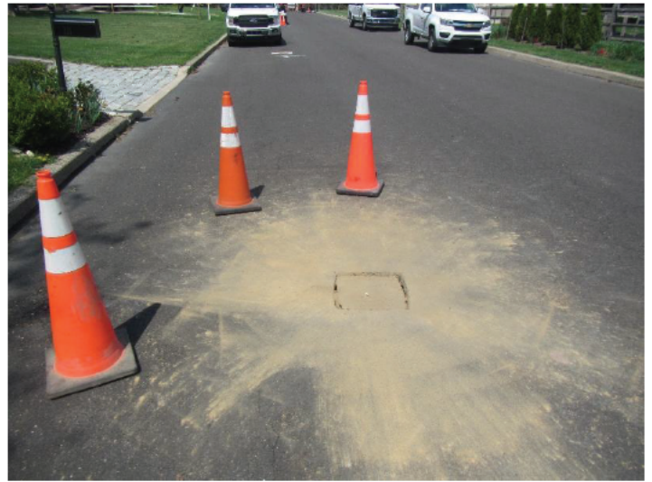
Well B location after completion of hand clearing.
