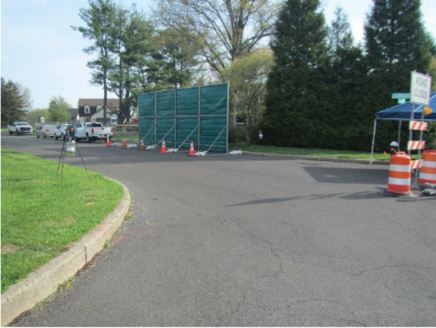
Sound barrier and road closure at intersection of Glenwood Drive and Walker Road.
