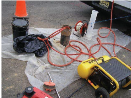
Photo 1: Pumping of Well-B Source: Olivia Budnovitch, 4/22/26
