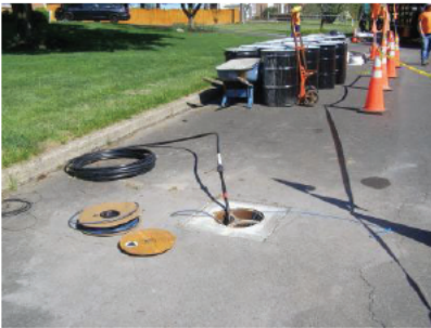
Inserted pump in monitoring well Well C on Glenwood Drive 4-27-26 @ 10:12
