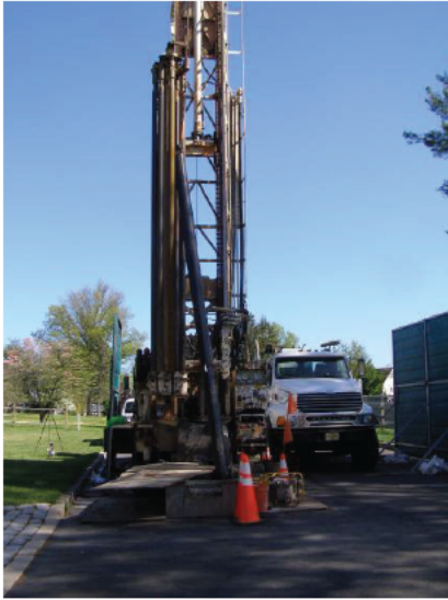
Drill rig over monitoring well MW-18DD 4-27-26 @ 9:18
