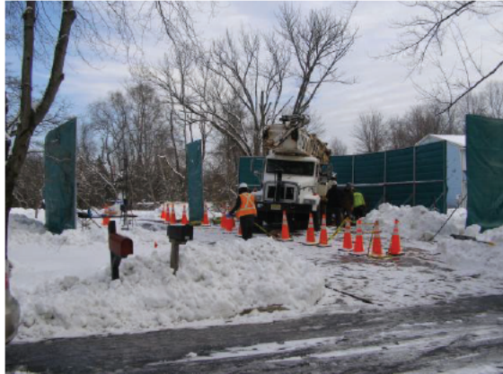
Drill Setup to install monitoring well MW-14D 2-2-26 @ 9:52
