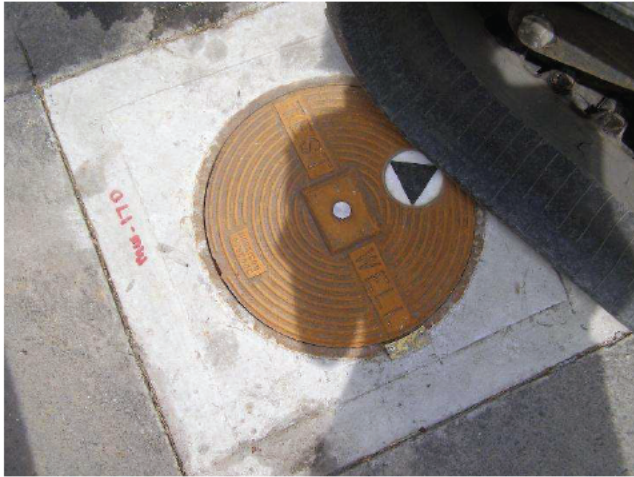
Photo 3: Flush mounting of MW-17DD
