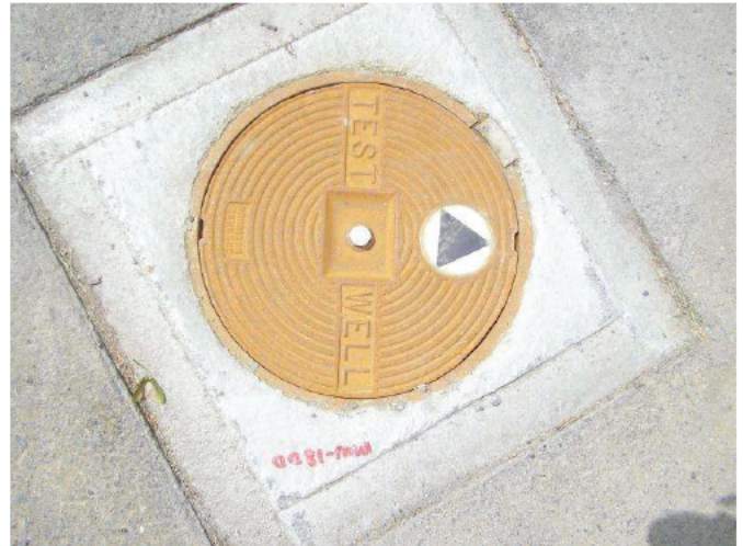
Photo 4: Flush mounting of MW-18DD
