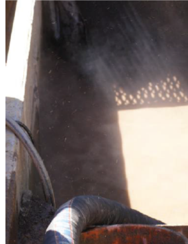
Vacuum truck hose collecting drilling and groundwater 5-4-26 @ 10:49
