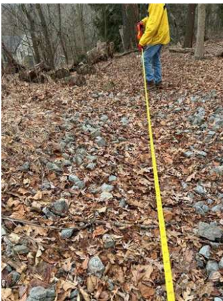
Photo 8: Measurement of riprap apron downgradient of rumble pad. (1-13-2026)
