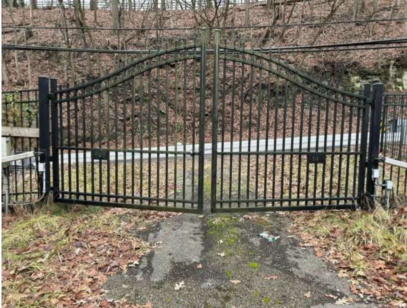
Photo 2: Gate at access road to site. (1-13-2026)
