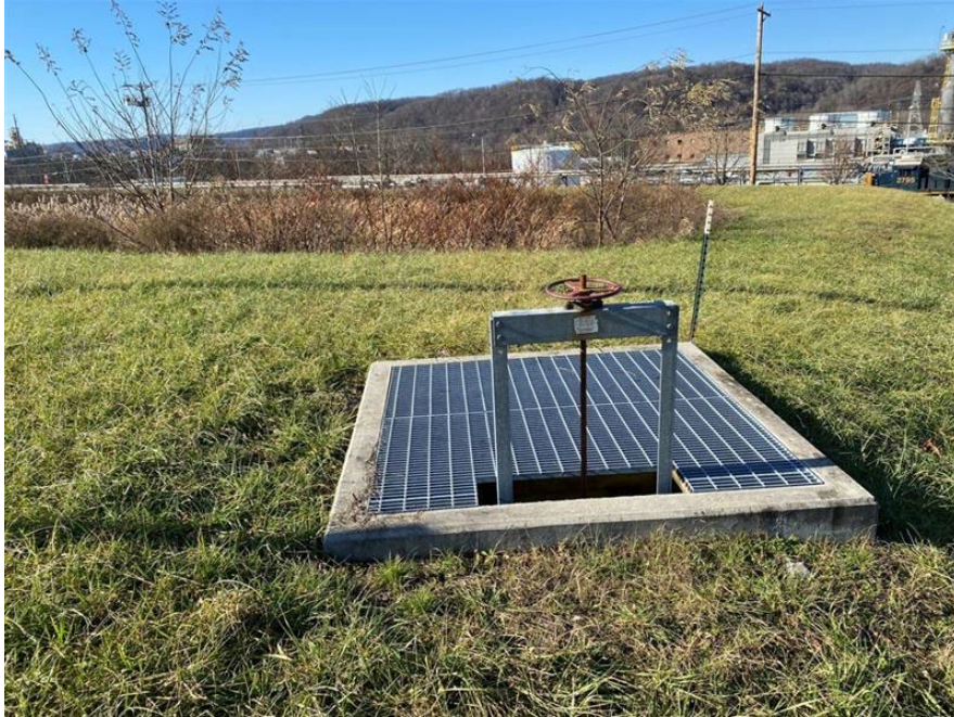
Photo 1 – Valve-controlled drainage box
