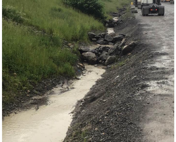
Trench to Outfall 016
