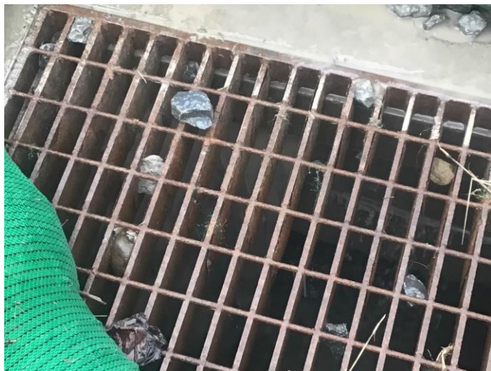
Grating to Outfall 016
