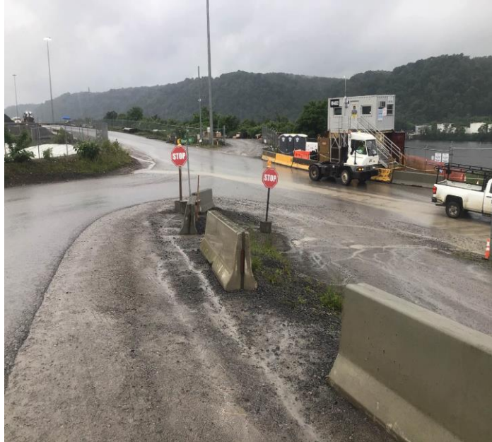
Road to Outfall 016
