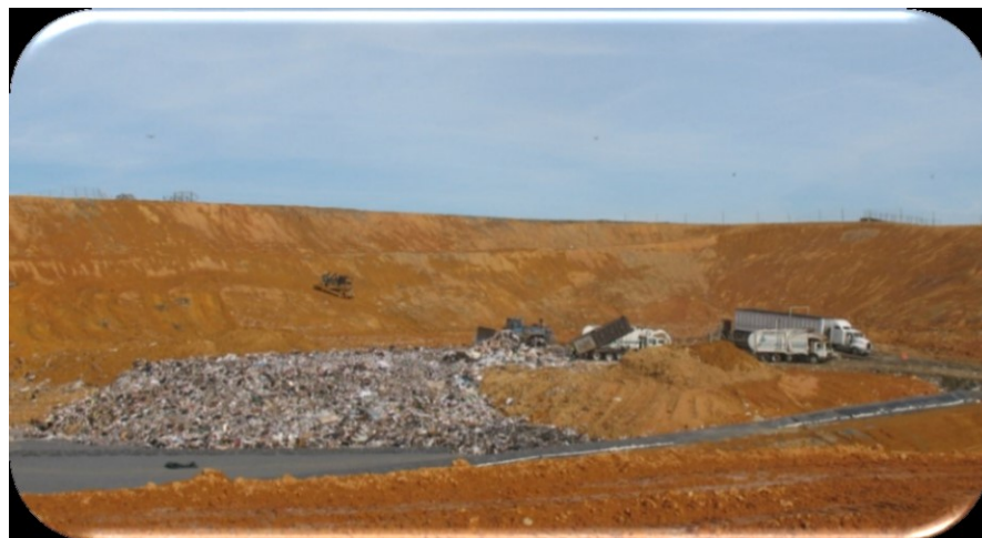
Mountain View Landfill face/dump area
