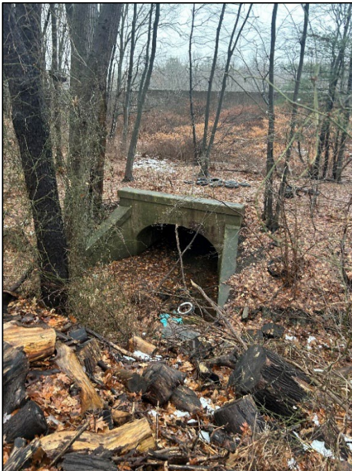
Old rail grade and bridge
