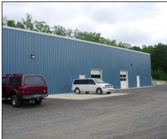
Figure 2 South Side of Building
