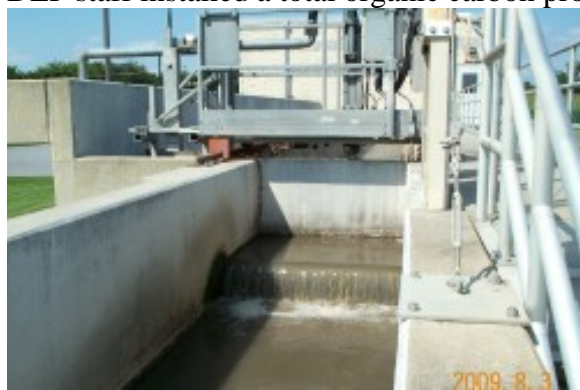
Figure 3.3: Inflow Channel after Grit Removal
