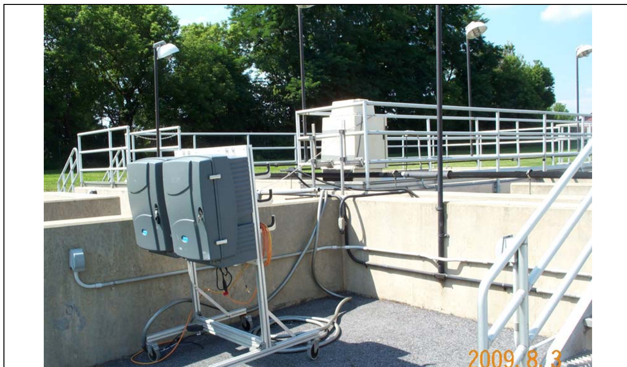
Figure H-3: Effluent monitoring equipment (Amtax NH 3 -N and Phosphax PO 4 -P)
