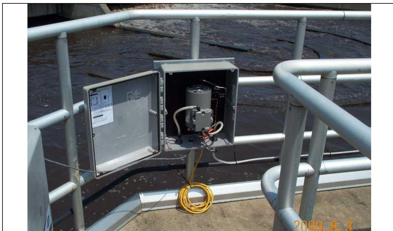
Figure H-5: Air-sparging compressor and drive motor for Ammonium ion probe.
