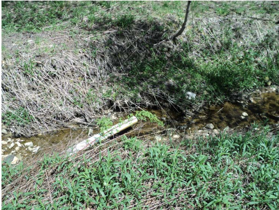
Figure F.7 Pump station overflow pipe to unt Wolf Run
