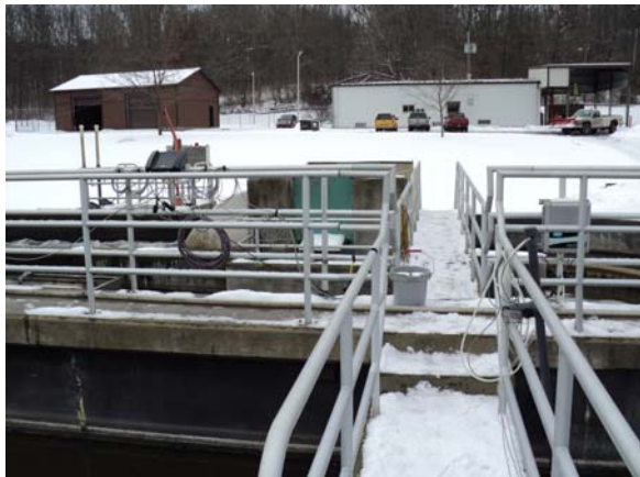
Figure F.3: Ammonium and Air Compressor, East Ditch
