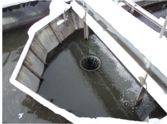
Figure F.8: Discharge end of boat clarifier
