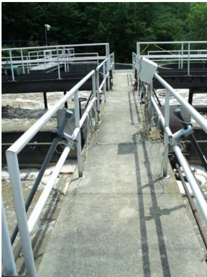
Figure E.1 Locations of ORP probes and SC1000
