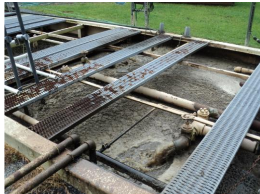
Figure C.2 Locations of ORP and DO probes in the anoxic tank
