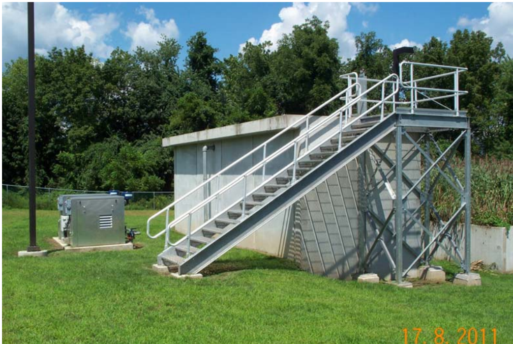
Figure G-2: Portland Aerobic Digester with Reed Beds to right.
