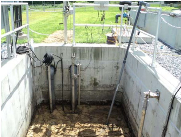
Figure G-18: Anoxic Tank Instrument Mounts
