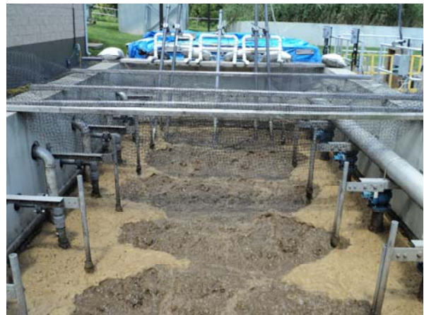
Figure G-15: Hach Probe Mounts in MBR 2
