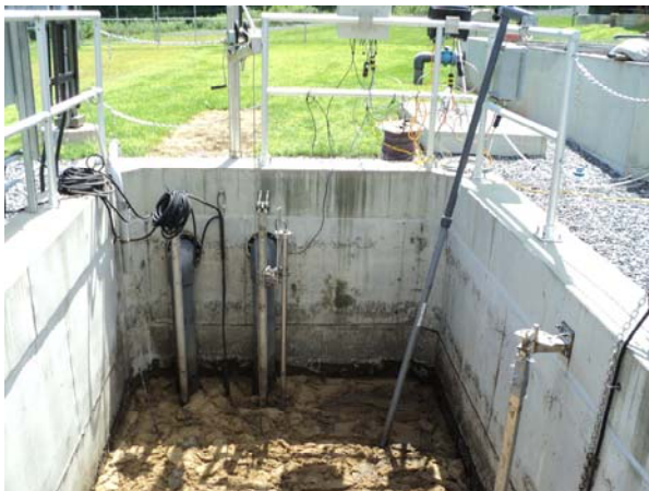
Figure G-14: Anoxic Tank Instrument Mounts
