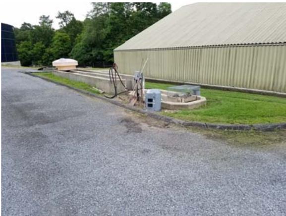
Influent channel w/ 24-hr Composite Sampler on loan
