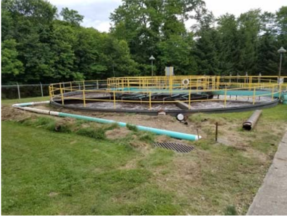
Unit 1 Reactor Conversion
