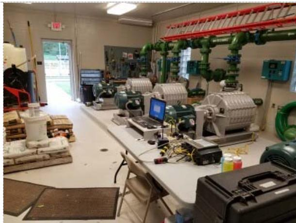
Centrifugal Blowers & DEP Monitoring Network. At left are the chemical feed system, with a work area in the far right corner.
