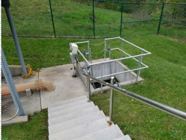
Effluent Balance Tank w/ Nutrient Probes : DEP had installed NO3-N and Ammonium ISE probes and added pH and DO for continuous monitoring. Shortly later, facility staff installed DO and pH monitoring probes that are tied to the facility SCADA system.
