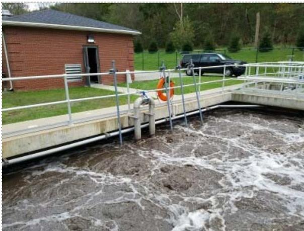
DEP Rail-mounted Immersion Probes: pH, DO, ORP, and MLSS
