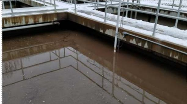
View of aeration tank during anoxic mixing phase: two new grinder pumps were installed at opposite ends of the tank, creating a whirlpool swirl of mixing during anoxic periods. Doing this kept the facultative bacteria in contact with both food (organic carbon in the wastewater) and nitrate ion in solution, the backup source of oxygen for cellular respiration.
