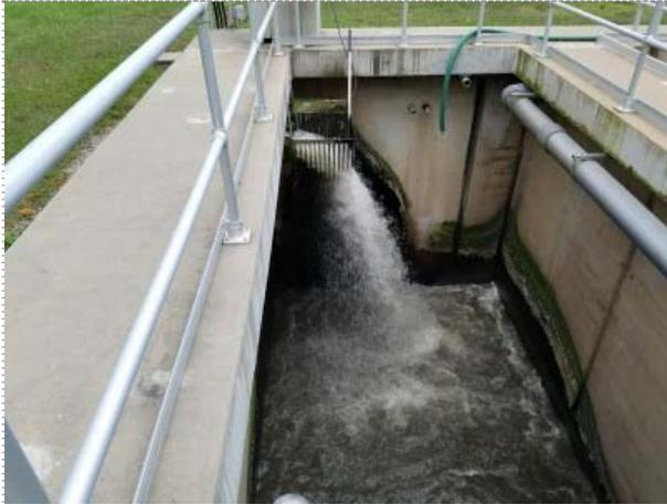
Equalization Tank & Bar Rack: equalization tank level should be maintained high enough to provide flow and load attenuation without endangering its capacity limit. The bar rack is not suited for a BNR facility, although it was adequate for extended aeration.
