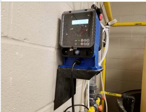
New metering pump used to feed  $Mg(OH)_2$  slurry
