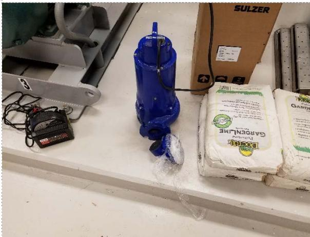
One of two new 230-volt grinder pumps used for anoxic mixing in the aeration tank. Alterations to the discharge end of the pump assured that current in the aeration tank would be in the form of a clockwise swirl instead of a geyser.
