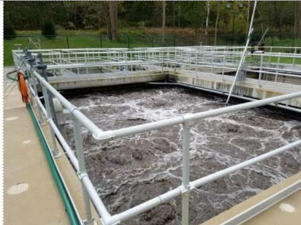
Aeration Tank with DO Sensor Probe at Upper Right and WTE probes at left. The DO sensor controls aeration blower valves to regulate oxygen content.
