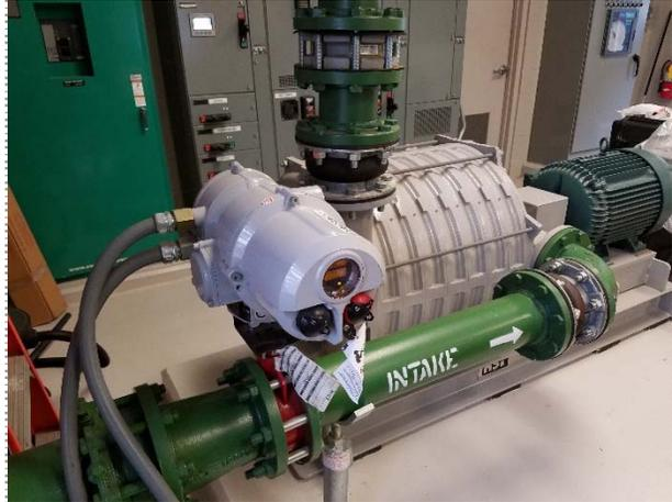
Intake valve regulator on centrifugal blower: Because centrifugal blowers are incompatible with variable frequency drives and operate at constant rpm, the intake valve is throttled to regulate air flow, supervised by dissolved oxygen residual in the aeration tank.
