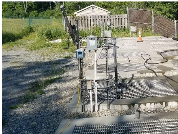
Post-WTE nitrate & D.O. probe at anoxic tank
