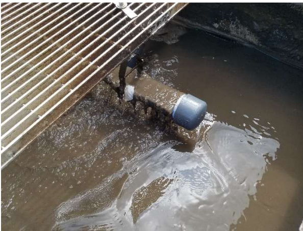
Modified recycle discharge
