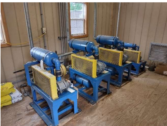
Rotary Lobe air compressors
