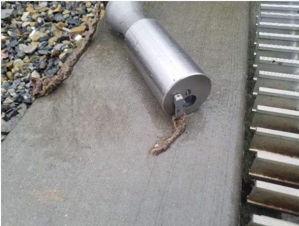
Rags collect on sensor probes
