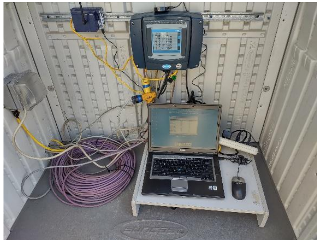
Figure B-7: Photo of WWTAP continuous monitoring network data logging, telemetry & display systems at the Curwensville WWTF.
