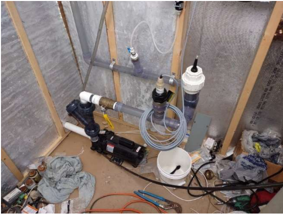
Effluent sampling and probe connections for continuous monitoring.
