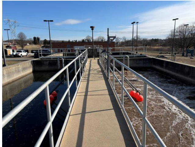
Figure B-4: Photo of continuous monitoring probe installation location in the WWTF SBR treatment units.
