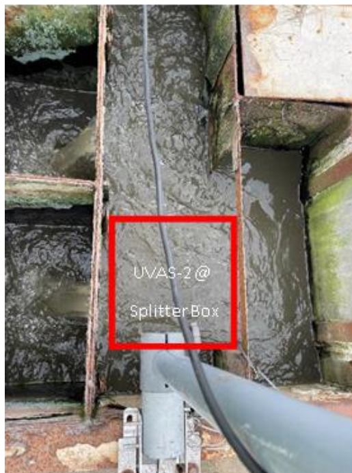
Figure 4: Photo of UVAS-2 continuous monitoring probe installation location (flow splitter box) in NESJMA WWTF from September 15 th through October 11 th , 2023 (end of study).
