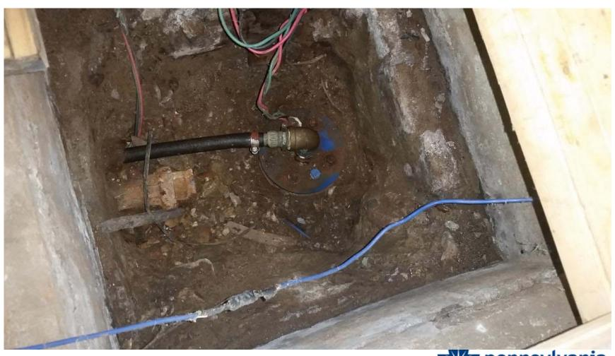
Lack of air gap for treatment drain lines
