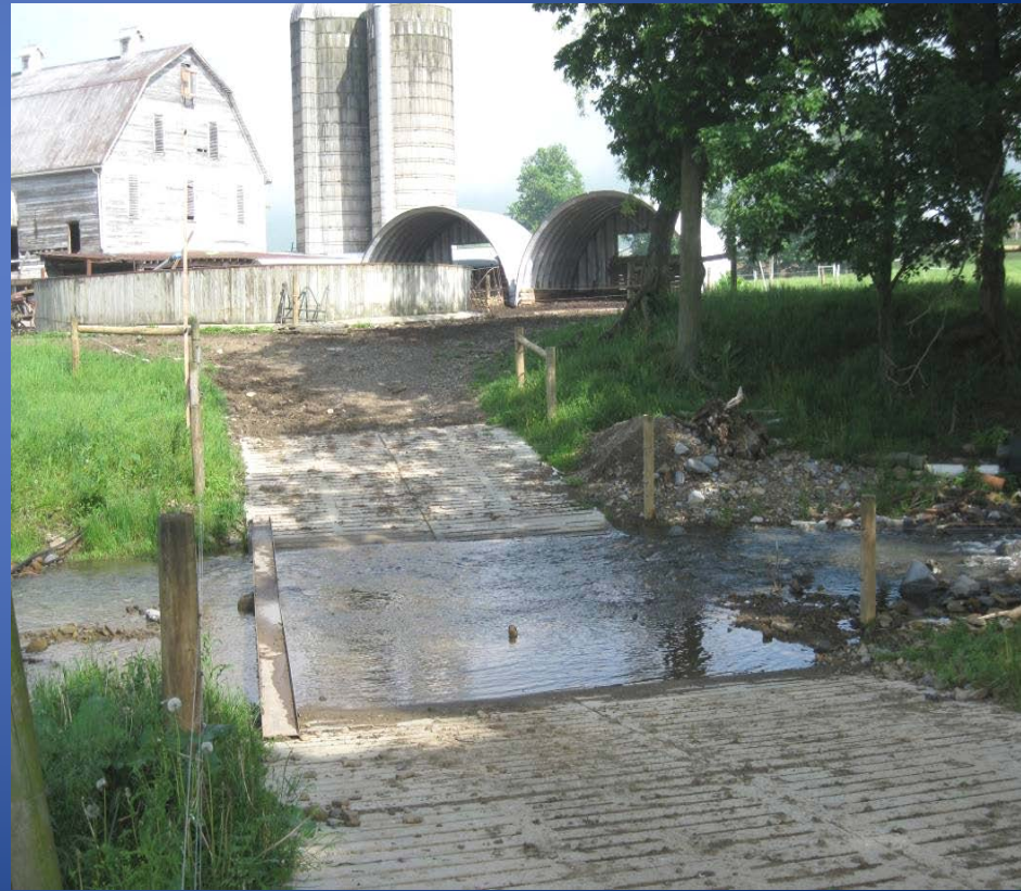
Stream Crossing – concrete hog slats
