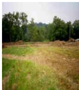
Construction in September 1998.
