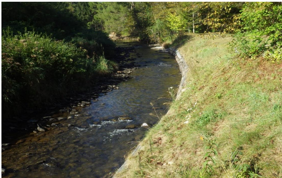
Previously completed stream bank stabilization project within Potter County
