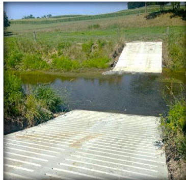
Figure 5 & 6. A new stream crossing and fencing system controls the cows' access to the stream, helping to reduce erosion and prevent sediment from entering the water.
