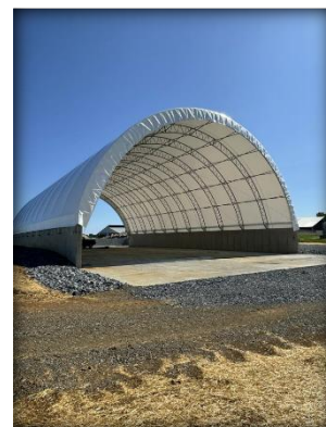
Figure 3. Hoop structure installed to address manure storage issues.
