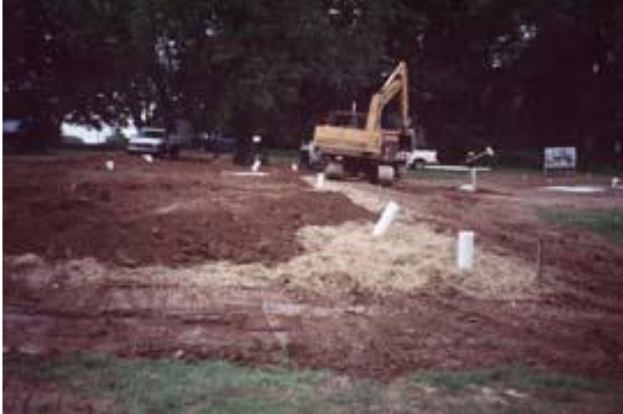
Soil cover being placed over beds.
