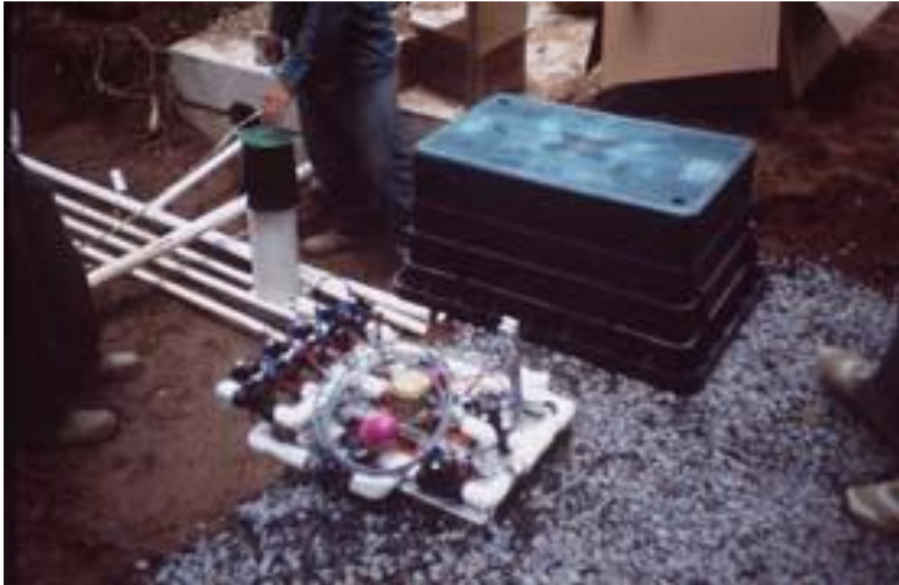
Controller being installed for trickle irrigation system.
