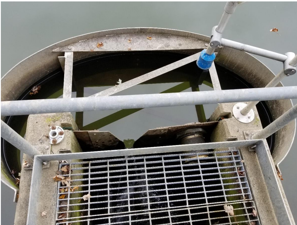
2 - Basin Outfall Structure & Sampling Point
