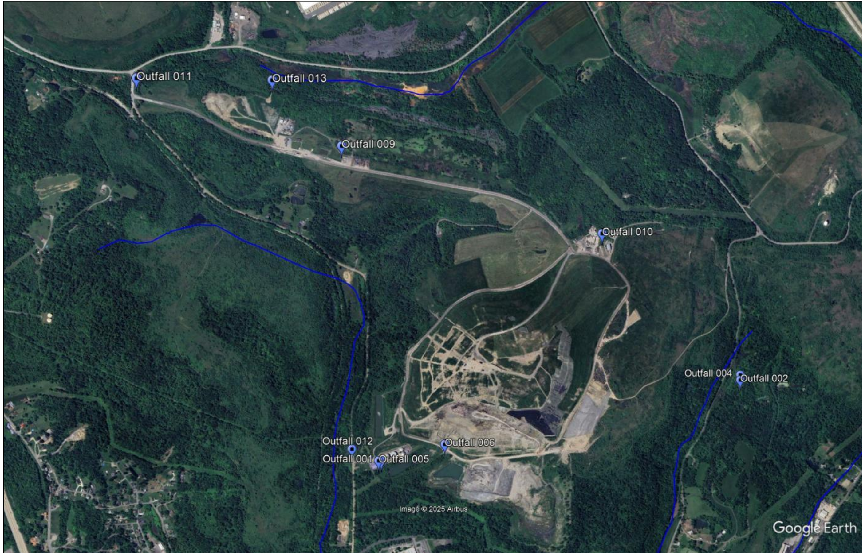
Image Source and Date: Google Earth Pro, June 1, 2025. Annotations by DEP.
