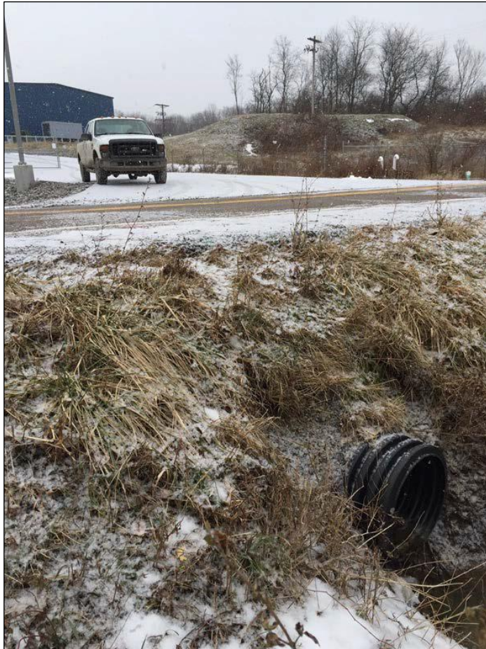
Figure 8. Outfall 012 and Partial Drainage Area View
