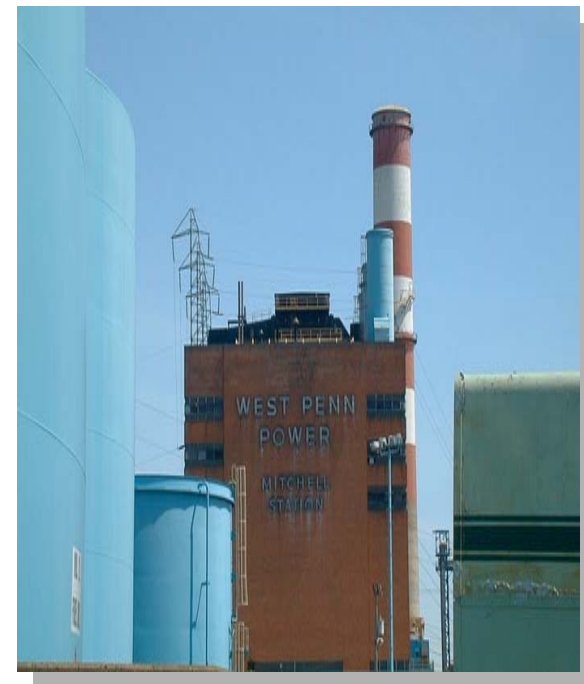
Allegheny Energy's Mitchell Station
