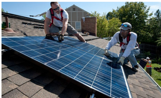
Residential solar installations can be perceived as commercial energy rates and increase utility costs. (Source: US Department of Energy)
