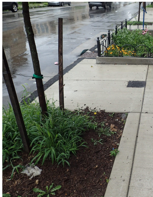
Stormwater can be absorbed and slowed by using garden beds in place of paved surfaces. (Philadelphia Water Department)
