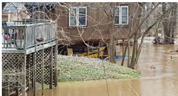
Flood damage is a cost associated with increased extreme weather events.
