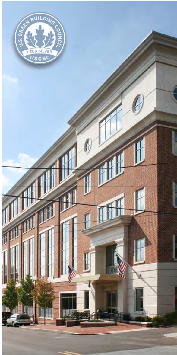
313 West Market Street is LEED Silver certified.
