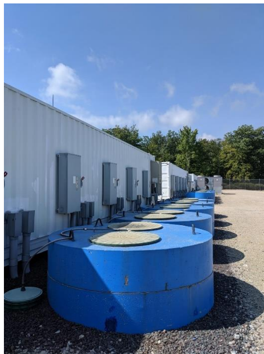
Figure 38. Flywheels in Hazle Township, PA
