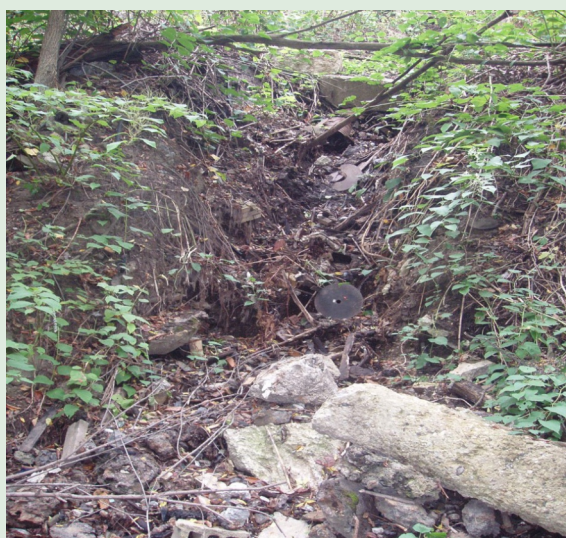
Foundry waste sand before the landslide and cleanup
