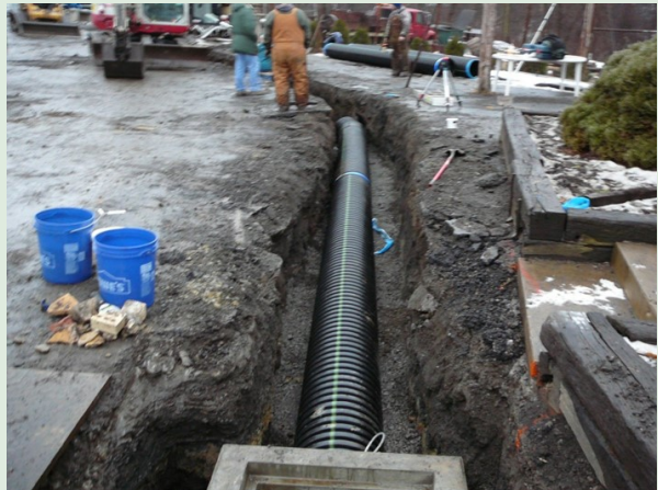
Storm water management during the cleanup
