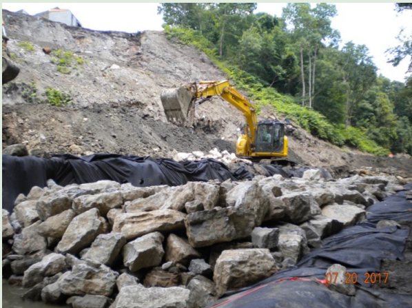
Slope stabilization during the cleanup
