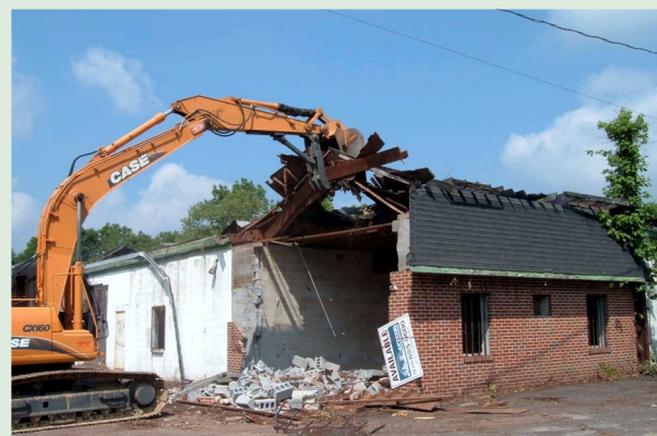
Demolition of the Plating Facility
