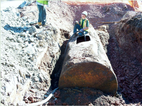
Emptying Underground Storage Tank
