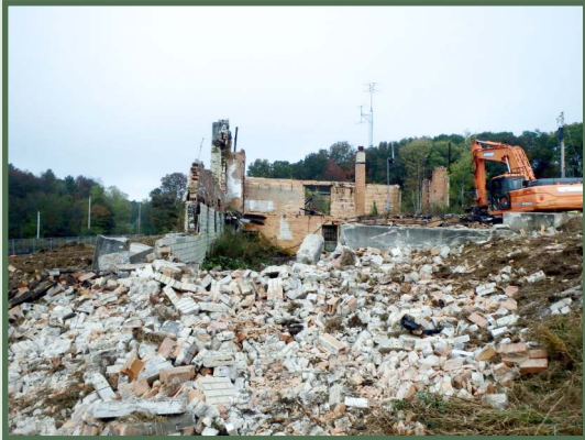
Demolition of the east side of building, October 2021.
