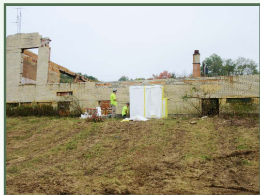
Bristol Environmental abating ACM on pipe insulation, October 2021.
