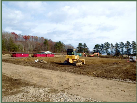
Grading in progress, November 2021.
