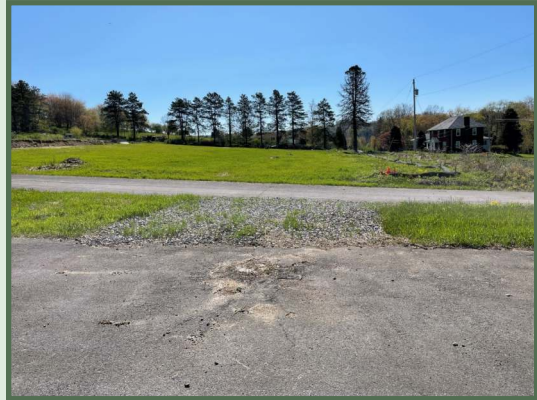
Vegetation growing, site complete May 2022.
