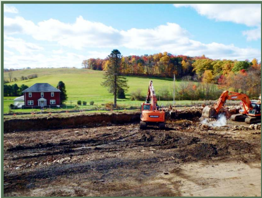
Building demolition process, November 2021.
