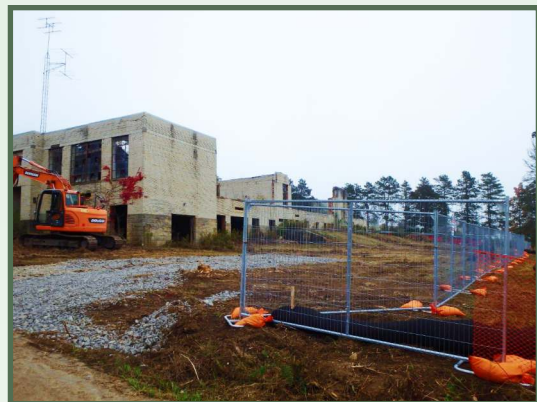
Vegetation cleared, erosion and sedimentation control in place, fence installed, October 2021.
