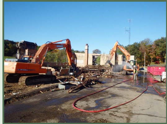
Application of water spray to control dust, October 2021.
