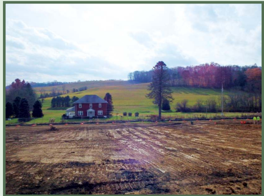
Site is graded and ready for seed mix, November 2021.
