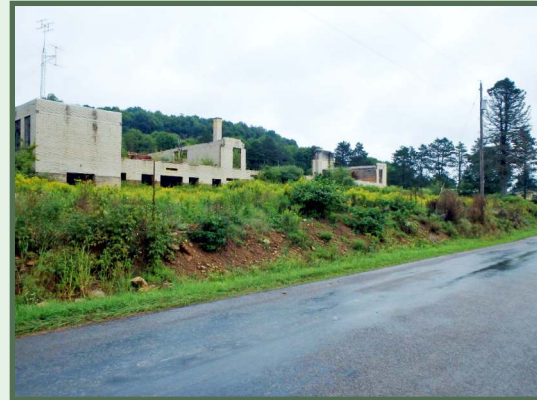
School building before demolition, August 2021.
