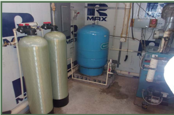
Impacted homes were supplied with whole house point-of-entry treatment systems with a primary and secondary carbon treatment vessel.
