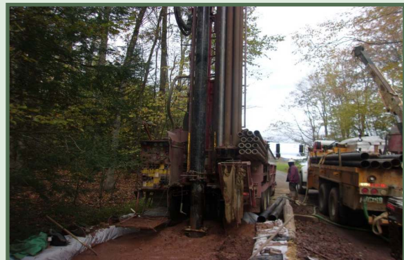
Installation of one of five groundwater monitoring wells.
