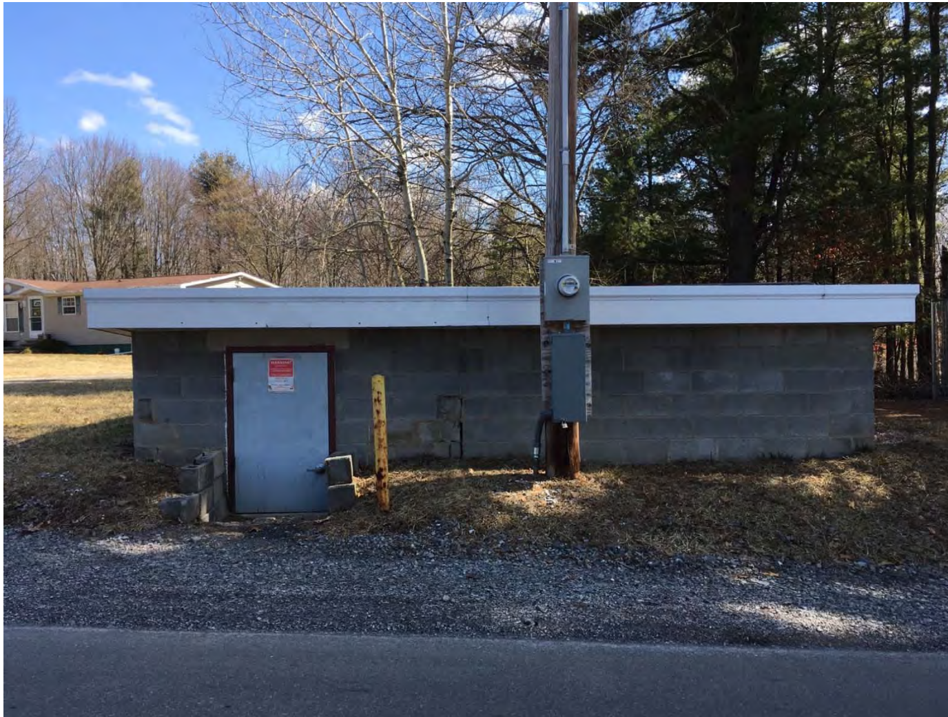
Existing Pump Station
