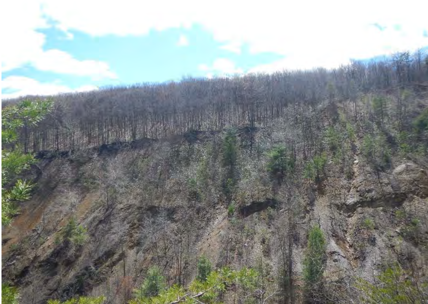
AML Feature 3233-01: Looking north at the Dangerous Highwall
