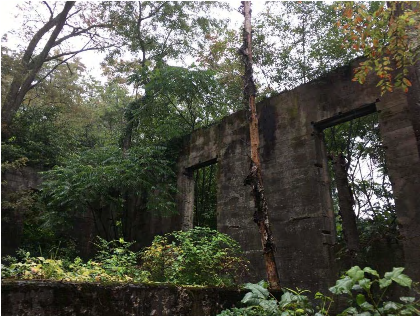
AML Feature 3233-22: Looking southeast at the building to be demolished
