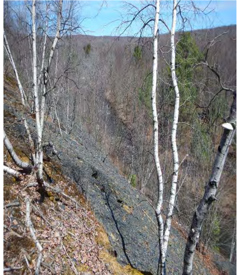
Dangerous Pile & Embankment
