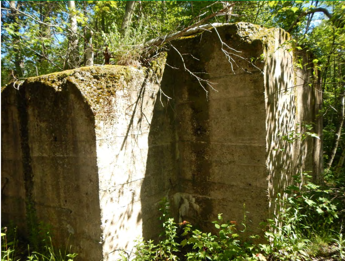
AML Feature 3756-09: Looking west at one of the equipment and facilities
