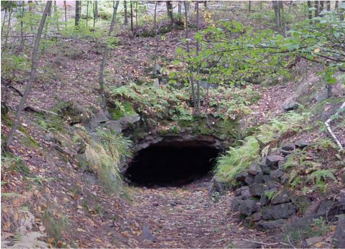
Photo 3: Abandoned mine opening where a bat-friendly gate will be installed.
