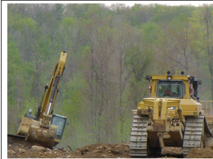
Haul Road Construction on Refuse Pile No.1
