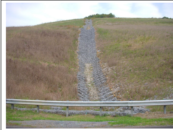
Gabion Baskets, Channel No. 3 on Refuse Pile No. 1
