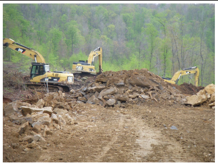
Haul Road Construction on Refuse Pile No. 1
