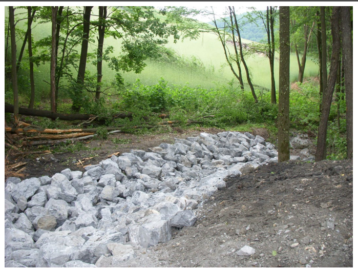
Channel No. 1 Grouted and Finished
