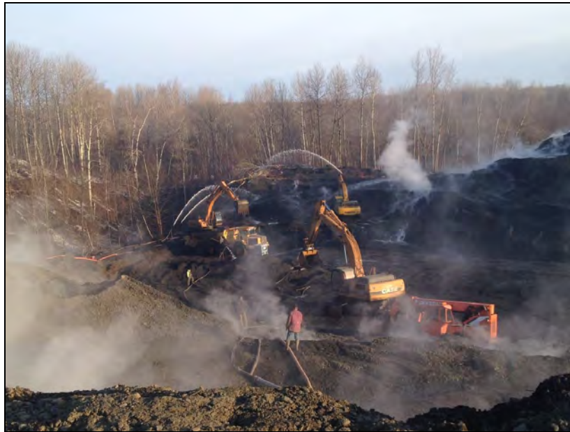
Contractor excavating burning material to install the cut off trench
