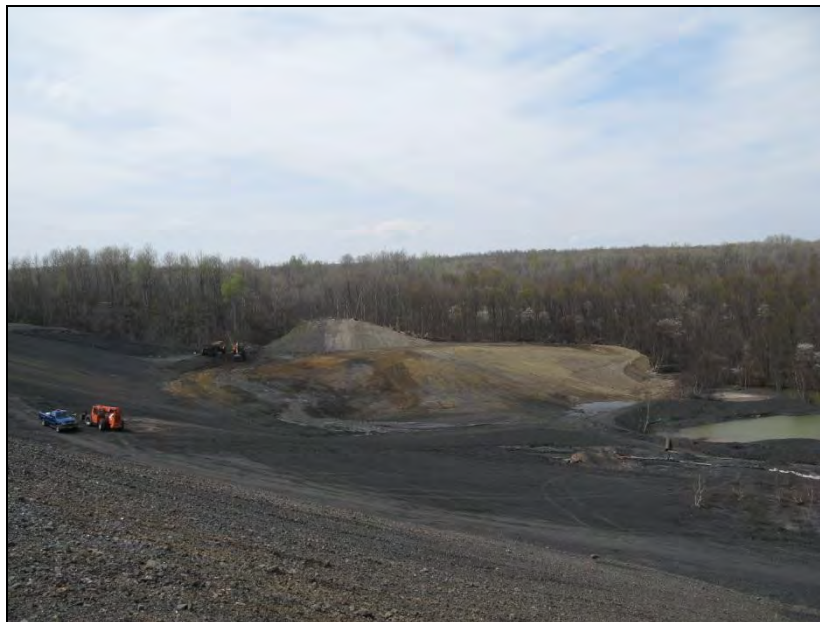
Fire Extinguished, project area being graded
