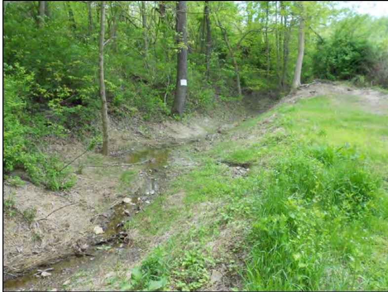
Post Construction - Completed Channel
