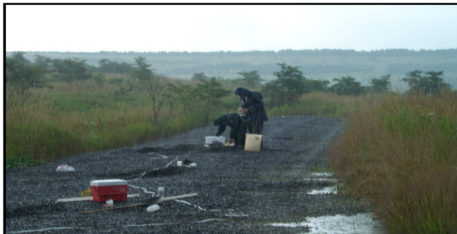
Figure 7.3. Typical Manganese Removal Bed
